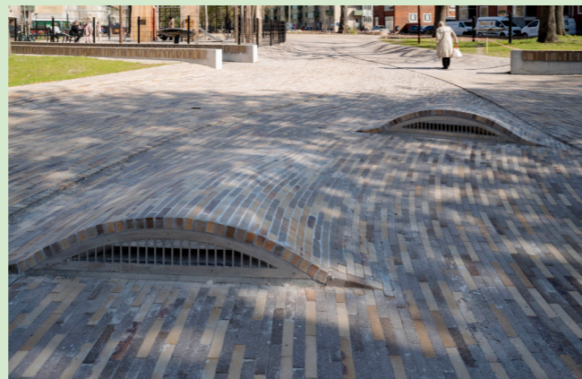
Water is transported in the open on the tiles through part of the axis.
