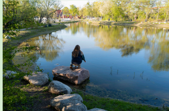
The rain water basin south of the axis adds additional capacity during heavy rain
